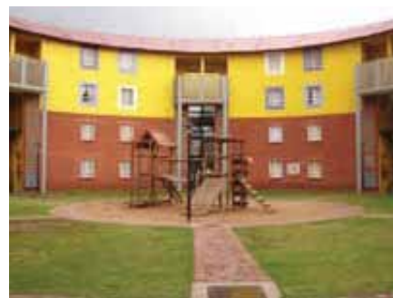
Brickfields Housing. Newtown, Johannesburg
